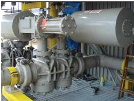
The valves illustrated are 12" class 2500 with hub ends. Criteria for selection: tight shut off, safety reliability and low maintenance.
