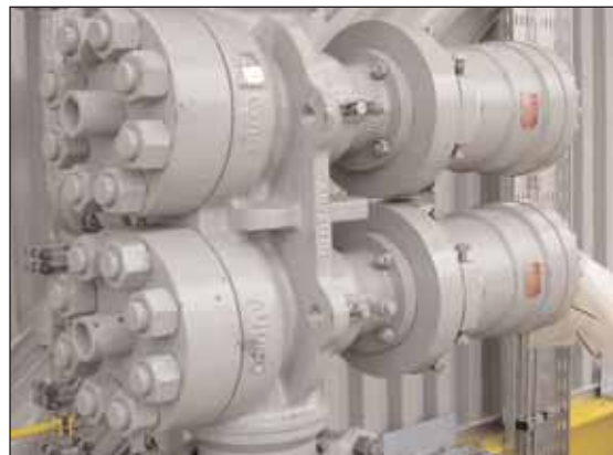
The valves illustrated are 12" class 2500 with hub ends. Criteria for selection: tight shut off, safety reliability and low maintenance.
